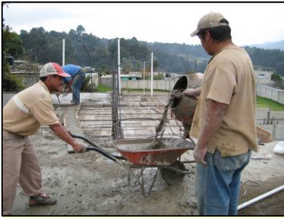
David & his crew pouring the roof over the family quarters
